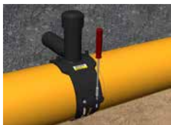
Figure C.34: Mounting the saddle
