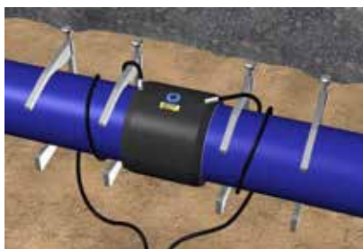
Figure C.17: Connecting the welding machine
