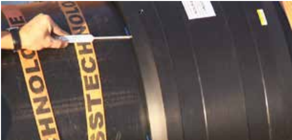
Figure C.26: Measuring the annular gap with the feeler gauge
