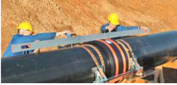
Figure C.22: Mounting of the clamping system and axially aligning of the pipe.
