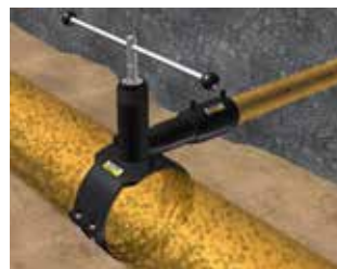
Figure C.36: Tapping of the pipe
