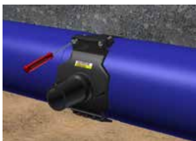
Figure C.31: Mounting the saddle
