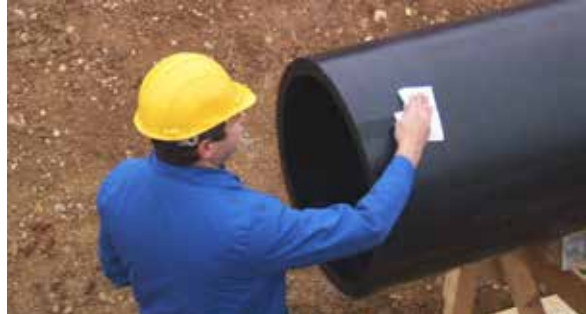
Figure C.21: Cleaning of the welding area
